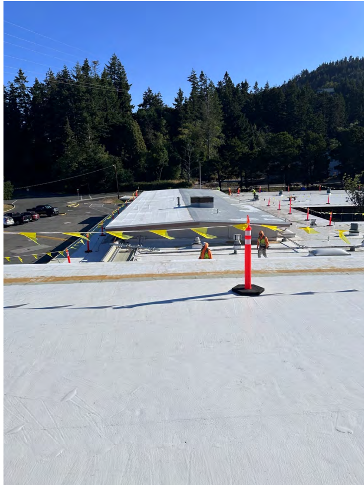
Progress Photo of Riley Creek Elementary Roofing Project
