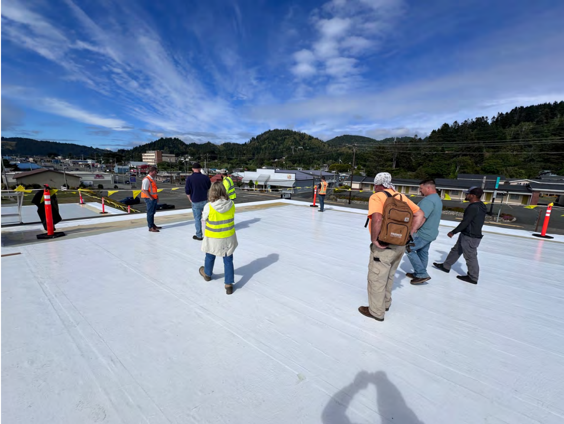
Gold Beach High School Post Roofing Project Review
