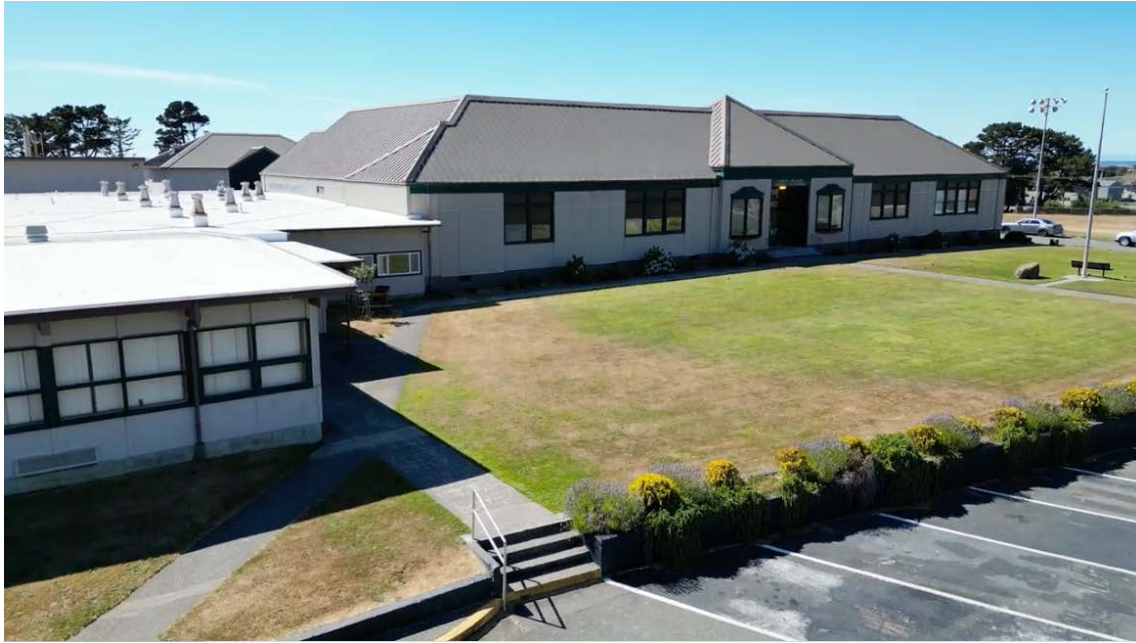
Gold Beach High School – Pre-Renovations
