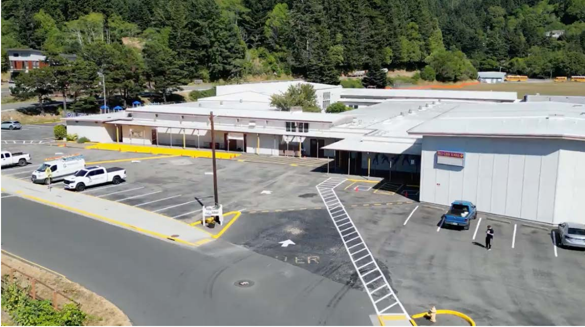
Riley Creek Elementary School – Pre-Renovations
