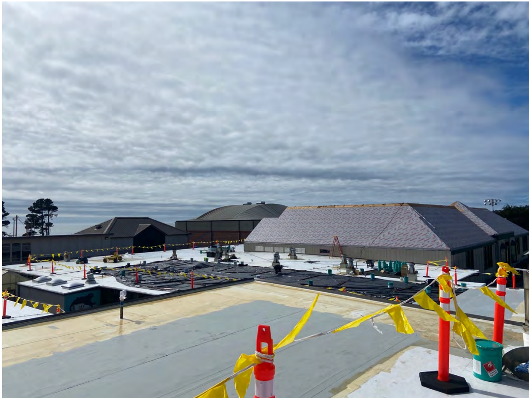
Gold Beach Junior/Senior High School Roofing Project
