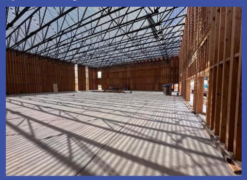
**Insulation and Roofing:** With the gym's walls framed and the roof structure completed, the next steps include adding insulation and continuing with roof installation.
