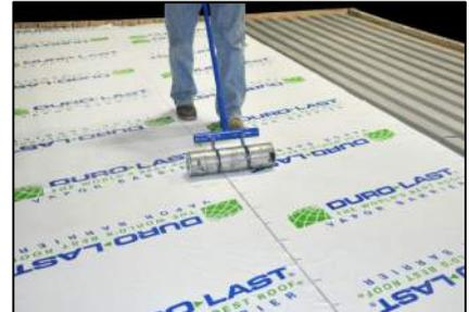
3. Install subsequent rolls of vapor barrier in the same way, taking care to overlap the longitudinal joints by 3 inches.
