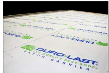
6. Once installation is complete, the Duro-Last Vapor Barrier temporarily protects against inclement weather. If not immediately covered, follow extra steps per 3a and 3b in the instructions above.
