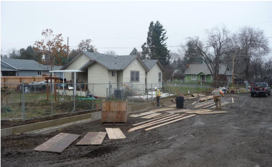
Footings for retaining walls were formed and poured in December
