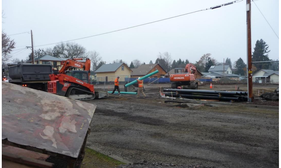
Work on the underground infrastructure at 2 nd Street is well underway
