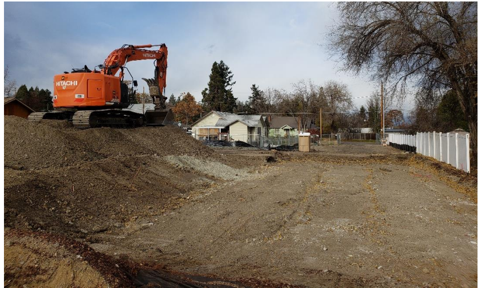
Demolition and excavation of the site was substantially complete in
