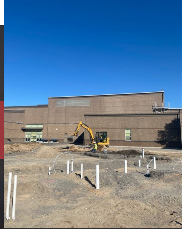
Plumbing utility stub ups getting installed and filled over.
