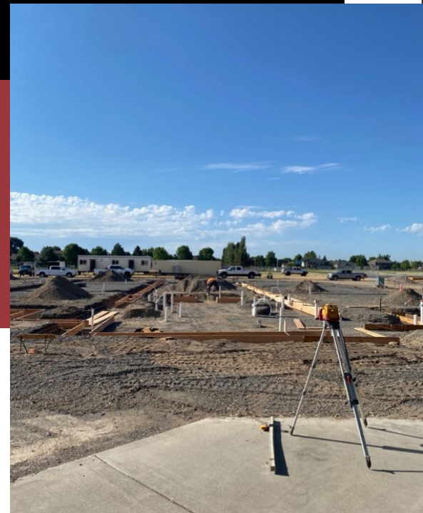
Fencing in place for Tom McCall students to access the field and footing casing being installed in preparation for concrete to be poured.
