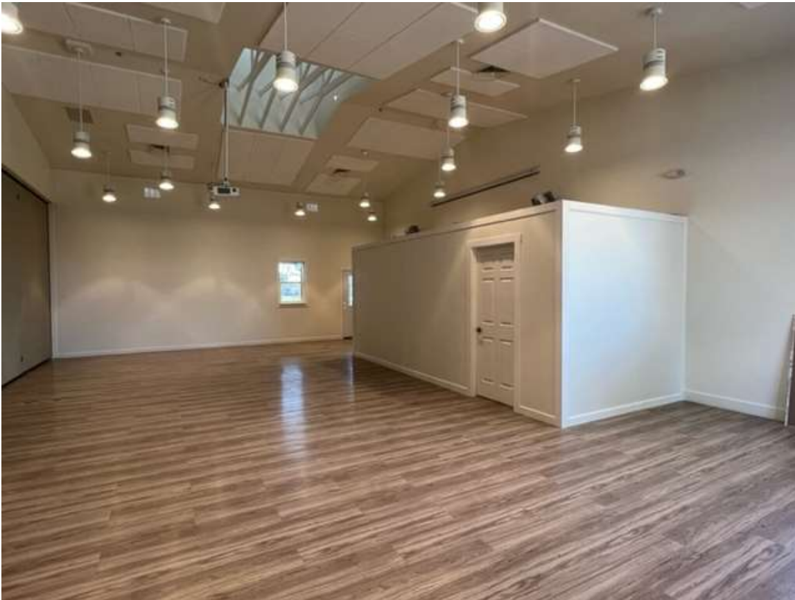
Public Works Superintendent Matias Mendez and crew completed the temporary office renovations for the police department storefront and locker room that saved the city significant costs and time.
